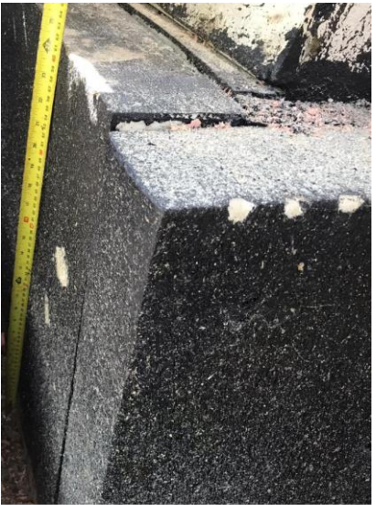
Walls below DPM to foundations XPS (expanded polystyrene)
