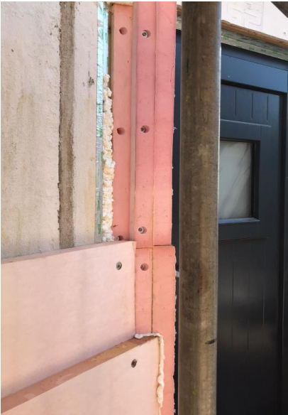
EWI, some IWI and new roof phenolic foam
